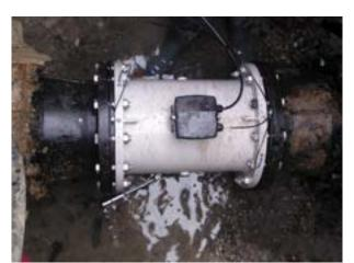
To ensure water bills are fair, and to reduce the need for verification, the MAG8 000 CT measures usage precisely and cost effectively with:
